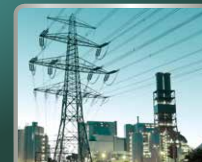
Power plant construction and maintenance
