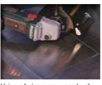
Using a "criss-cross procedure" systematically prepare the surface using the inflatable expansion roller fitted with the Pyramid sanding belts. Steadily work through the grits, A 45, A 30, A 16, A 06 one after the other with the burnishing machine on full speed setting 6\*.
